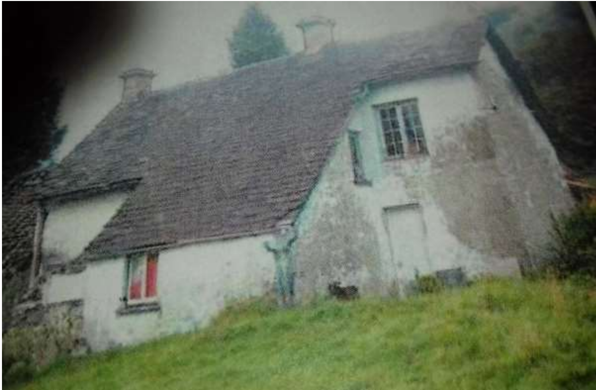
Figure 5: The rear of Ty'n y Ffynnon farmhouse showing the dairy
