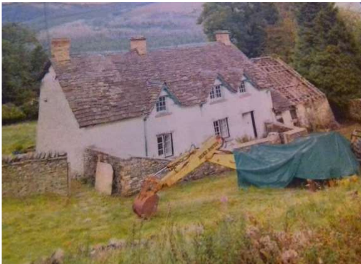
Figure 2: Ty'n y Ffynnon farmhouse prior to modernisation in the early 2000s
