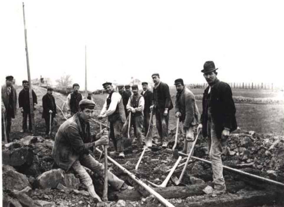
Figure 8: Platelayers at work on the Mountsorrel branch line in Leicestershire
