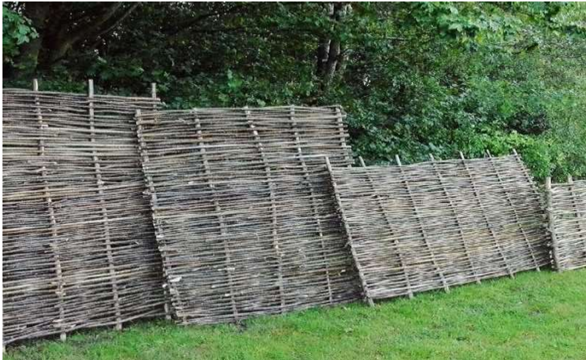
Fig 2 Woven greenwood hazel hurdle fence panels were once a common feature of rural life (unknown source)
