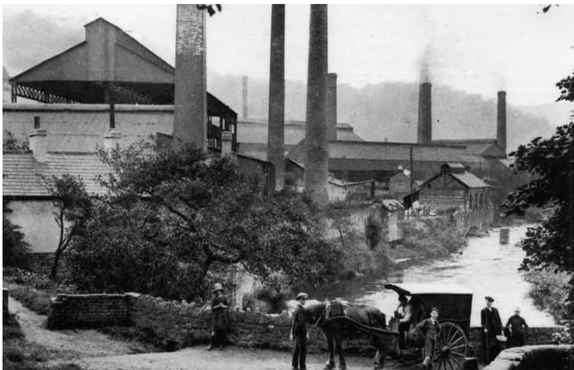
Fig. 16 Looking up the River Ebbw towards the Pontymister works from the Ochryth side of the Stoney Bridge.
