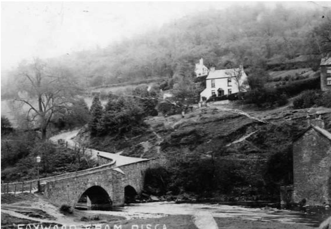
Fig 15 The Stoney Bridge at Pontymister. This would have been walked across regularly by generations of occupants of Ochryth including Polly Morgan on her way to and from the cottage at Penrhiw-gwial
