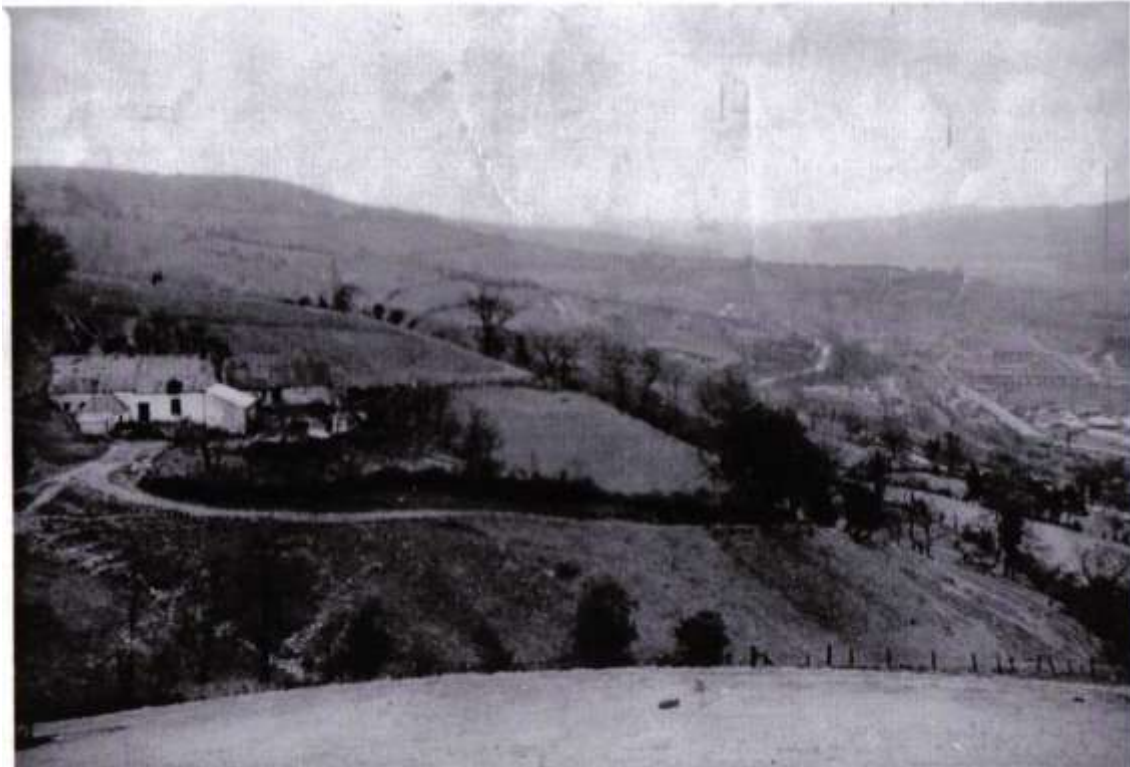
Fig. 9 A view of Cwmyr Uchaf dated 1947. This was taken from a field on the opposite side of the Cwmyr brook (Source: Risca Museum)
