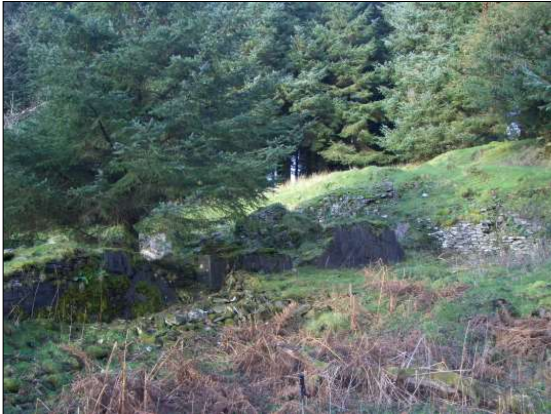
A sideways view of the longhouse with the cow house to the left and living accommodation uphill to the right. The two sections are separated by the entrance to the cross passage
