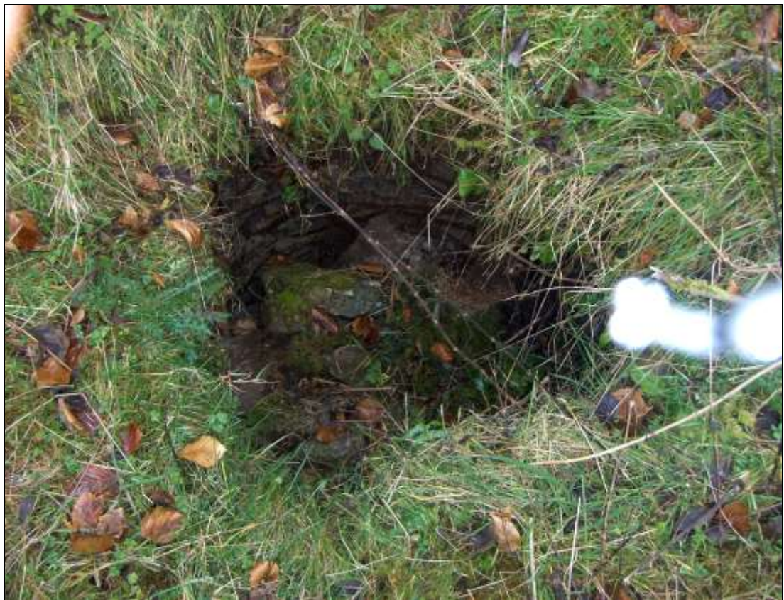
The remains of the well shaft. It was blocked up but now the infill is sinking fast.
