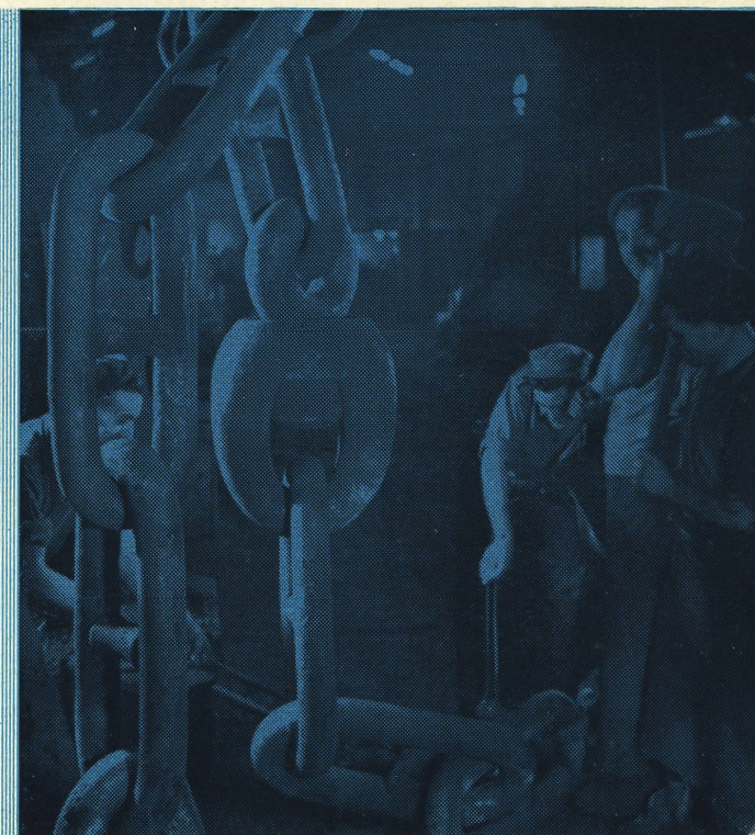
A number of links and a swivel of the 3\frac{1}{2} " wrought iron Mooring Chain for the Regent Oil Co. Ltd.'s mooring at Canvey Island, photographed in the Chainworks at Pontypridd.
