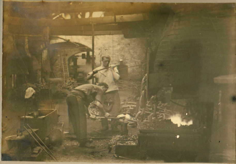
Chain Making (side welder)
