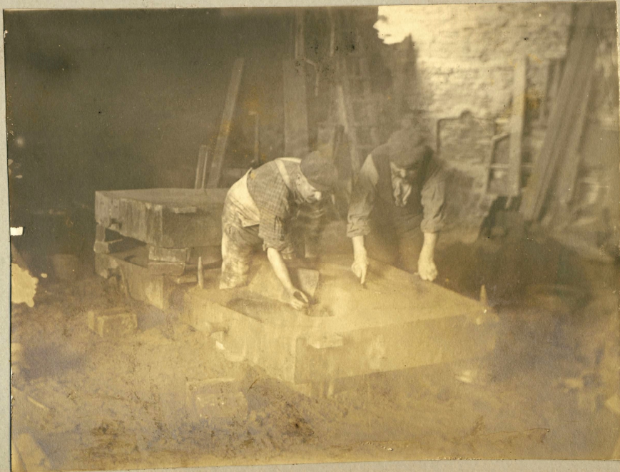
Showing method of Casting crew head on to a mooring screw.
